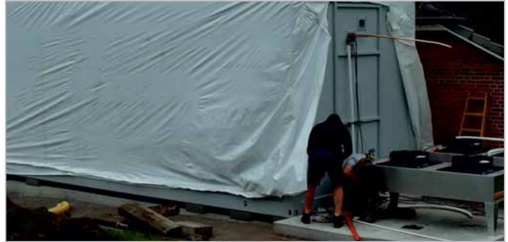
Installation of air conditioning systems with condensers
