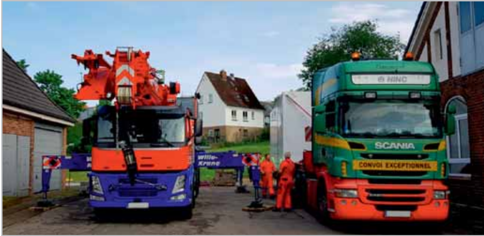
Unloading and placing on a concrete base
