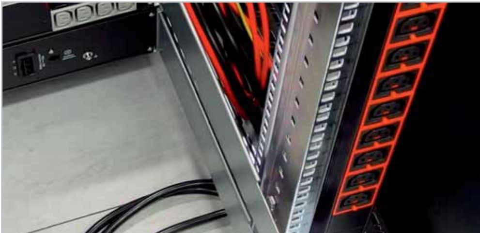
Installation of UPS & PDUs BPS2000
